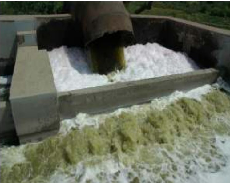
The so-called treated wastewater is used for irrigating 2500 hectares of land.
